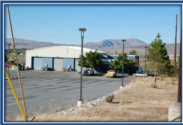
Kurt Svare Transportation Center (aka North Yard)
