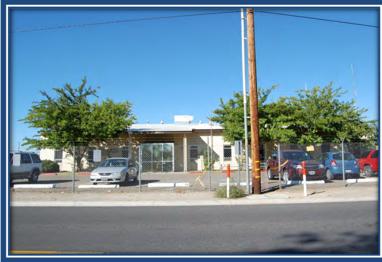
George Getto Transportation Center (aka Central Yard)
